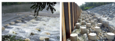
Diagrams and examples of rock chutes with staggered arrays of elements. (a) and (b) Diagrams of rock chutes with staggered arrays of elements. (c) rock chute at the Carénac weir on the Dordogne River. (d) fish pass at the weir for the ASF A7 highway over the Rubicon River
